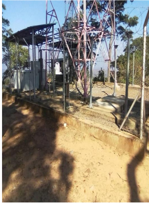
Figure 2: Airtel Tower in Thambani Forest Reserve
