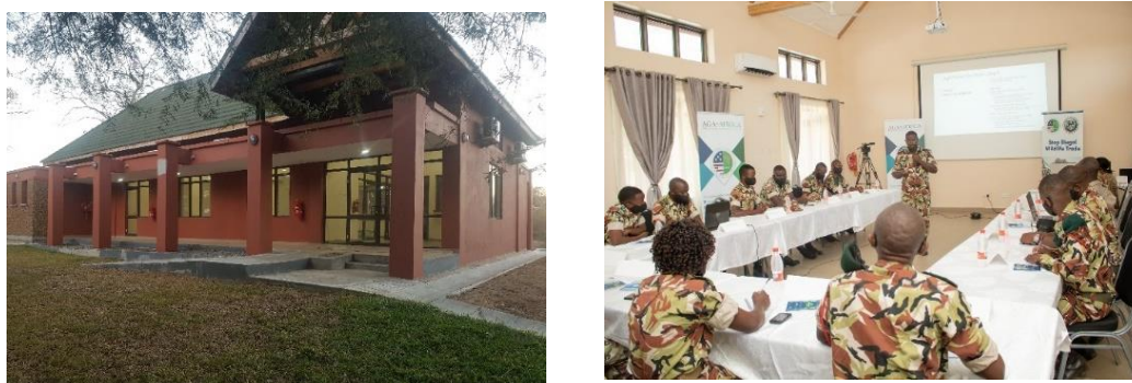
Figure 28: Photographs of the exterior view of the newly constructed Conference Centre at Nyala Lodge (a) and the rangers attending a training at the Conference in October, 2020 (b)
