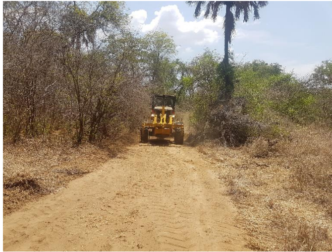
Figure 31: Photograph showing the road grading in Old Lengwe.
