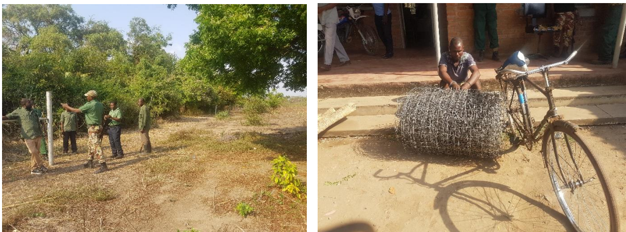
Figure 33: Photographs of the vandalised fence on Billiat Side, Ndakwera (left) and apprehended culprit (Right)
