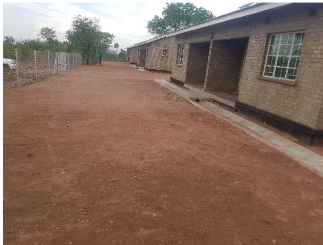
Figure 29: Newly constructed Jasi camp
