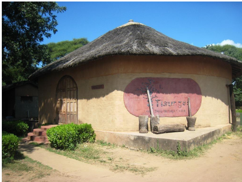
Figure 11: Photograph of the main Tisunge (museum) building at the entrance of Lengwe NP
